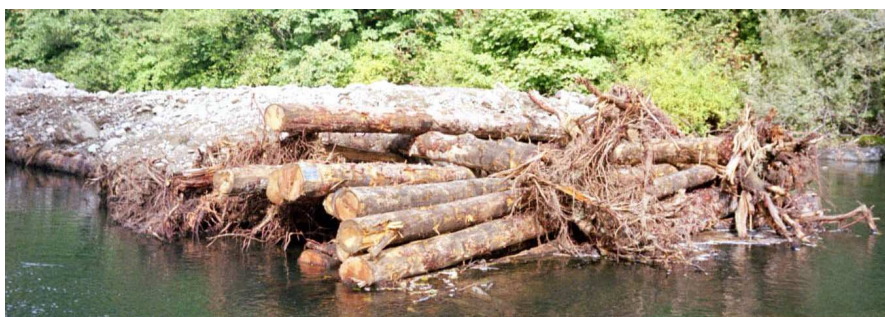
Obr. 2: ELJ na Green River (King County, Washington)
